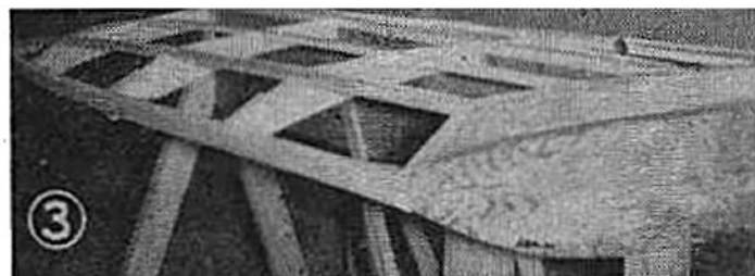
Note outer frame attached to the transom.
